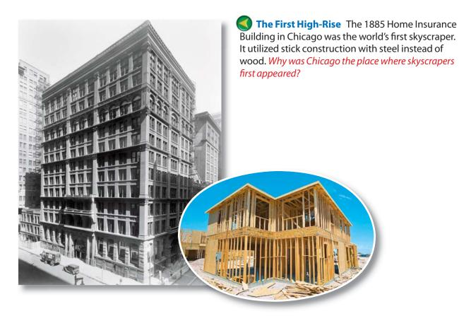
The frames went up quickly and provided both safe and strong dwellings. Almost all modern houses are still built this way. Even skyscrapers can be built with a type of stick construction that uses steel.
